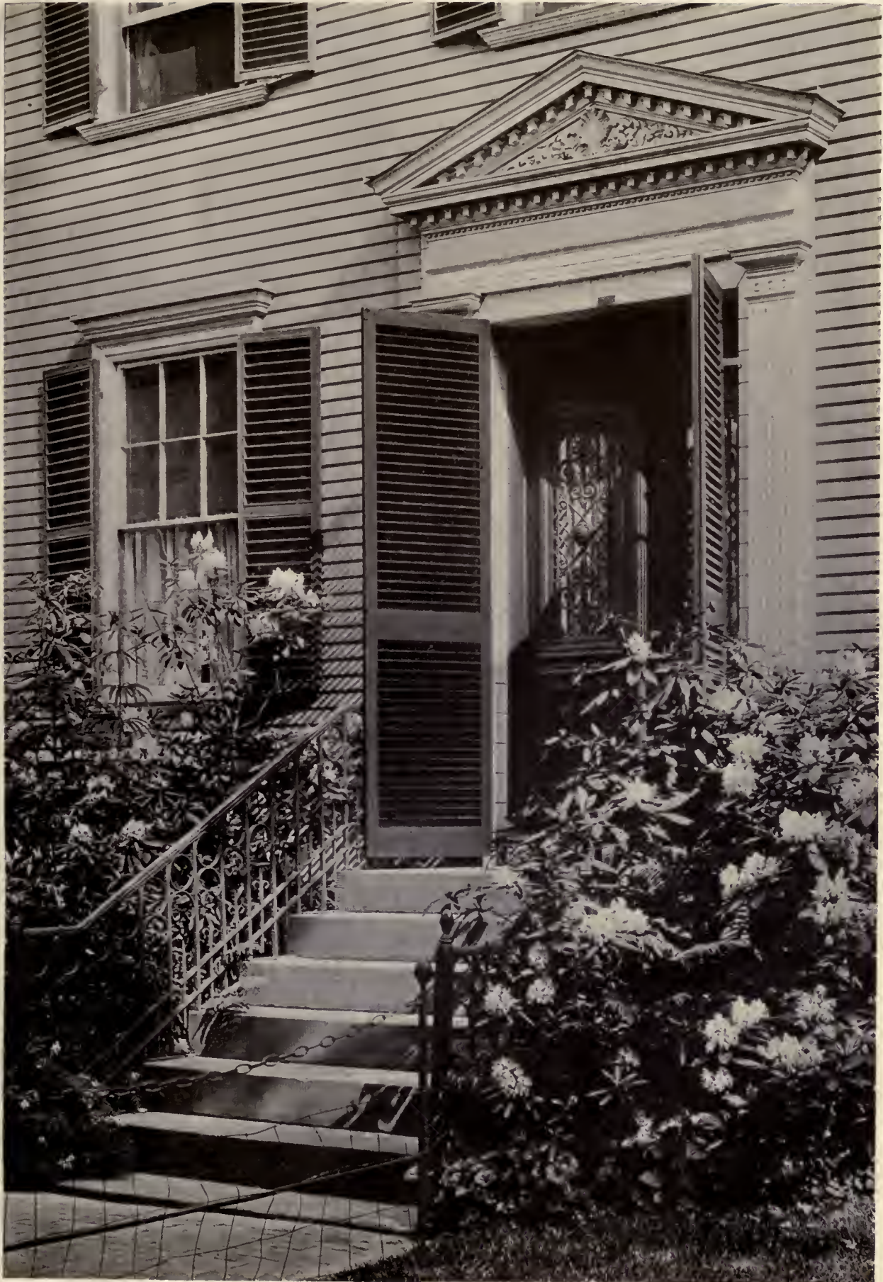
DOORWAY CABOT-ENDICOTT-LOW HOUSE, ESSEX STREET, SALEM, MASS. SAMUEL McINTIRE, ARCHITECT
